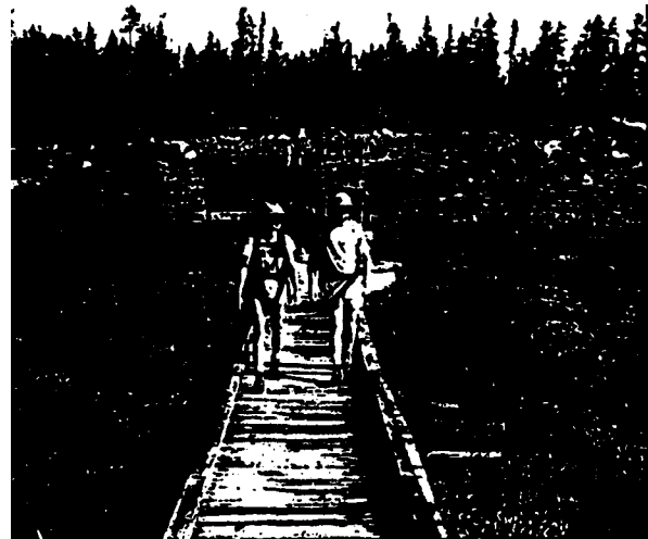
Figure 5.10 This elevated walkway separates hikers from the boggy soils underneath. (Photo by D. Cole.)
